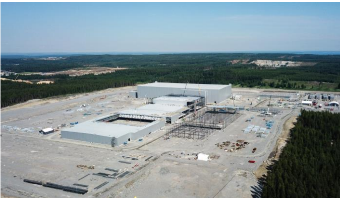
Northvolt Ett in Sweden, under construction
